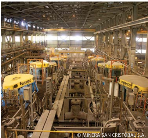
© MINERA SAN CRISTÓBAL S.A.
